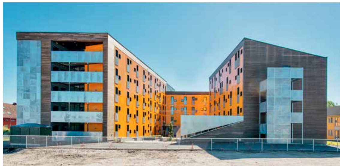
Orange is the signature colour of the Student Welfare Organisation in Østfold, so it was natural to use orange on the student housing complex in Fredrikstad.
