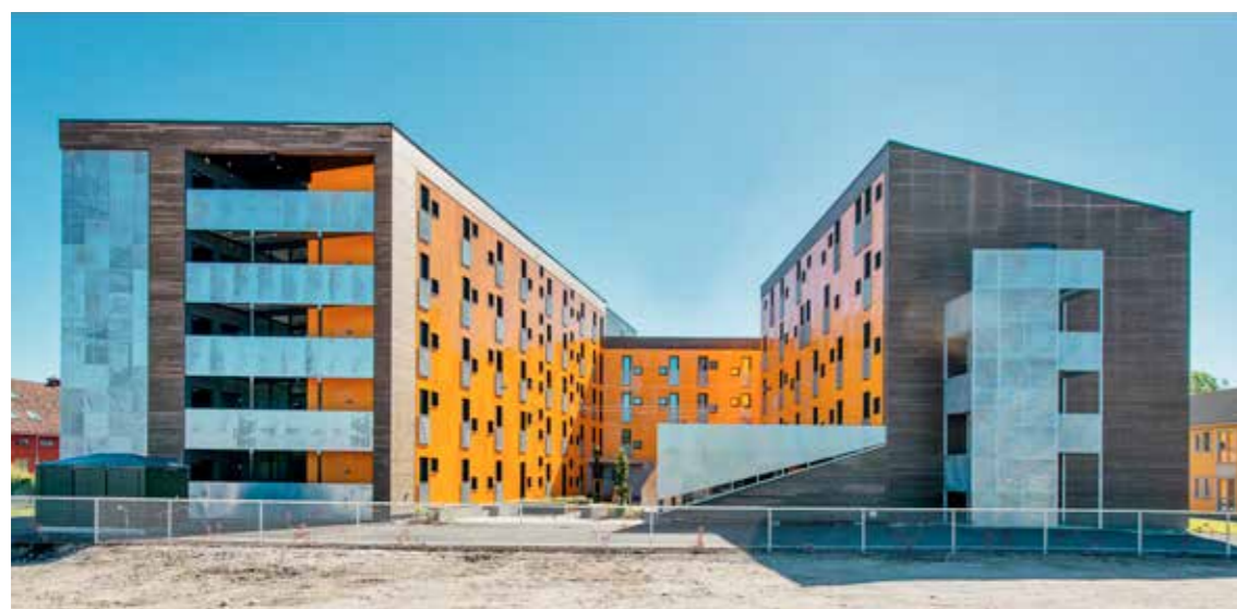
Orange is the signature colour of the Student Welfare Organisation in Østfold, so it was natural to use orange on the student housing complex in Fredrikstad.
